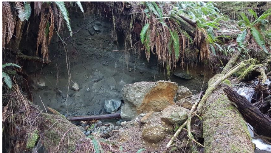
Photo 4 - Undercut bank in mid-section of Creek 3C with exposed gravelly subsoils
