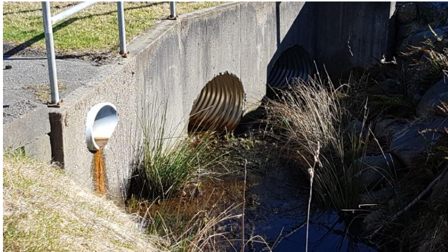
Photo 14 - Double 900mm CSP Pipe Arch Crossing of Kelsey Way
