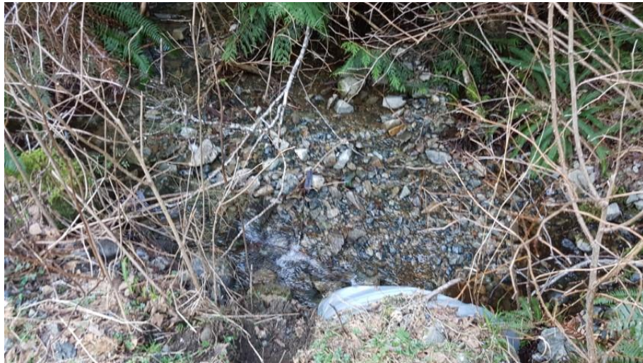
Photo 2 - Culvert outlet at Creek 3C crossing of M-Branch
