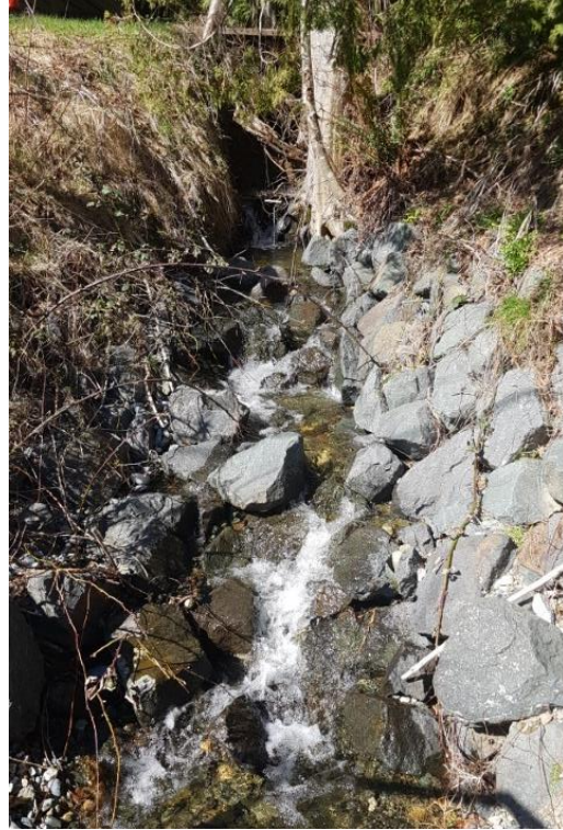
Photo 7 - Drainage ditch upstream of Headwall 1
