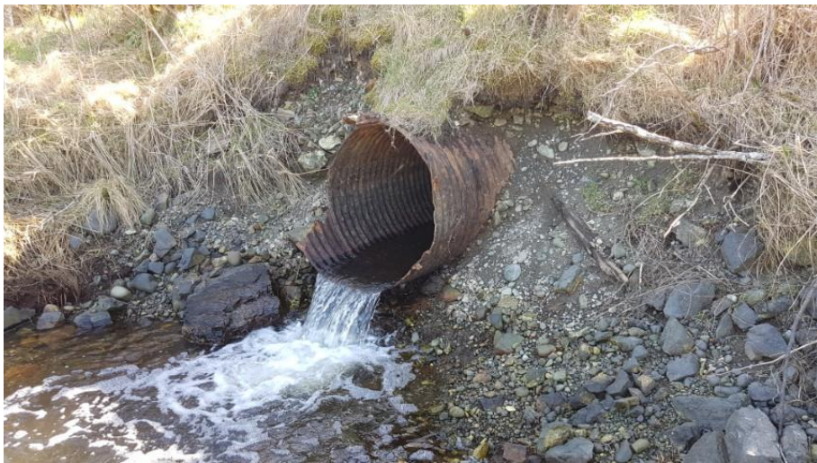
Photo 10 - 1050mm culvert outlet from storage pond to Salmon River estuary
