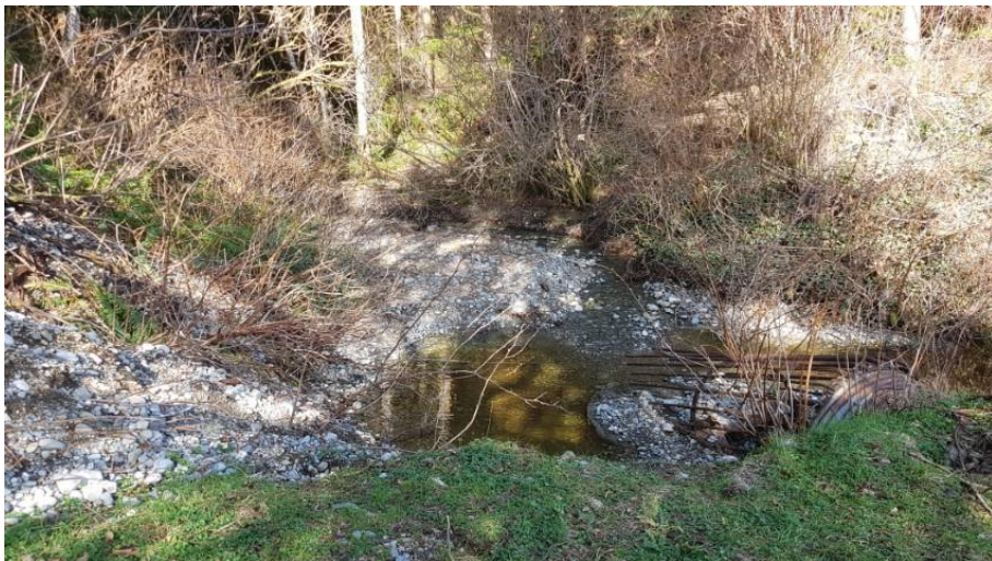
Photo 11 - Creek 3C inlet pipe/trashrack
