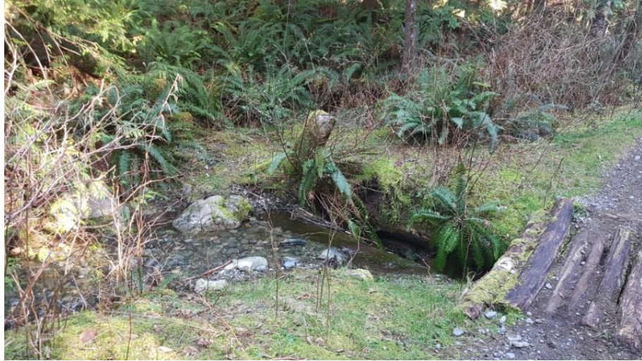
Photo 5 - Wooden log diversion structure for Creek 3A & 3B flows (water flows left to right under the trail)
