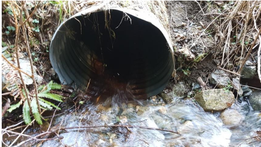
Photo 1 - Culvert inlet at Creek 3C crossing of M-Branch
