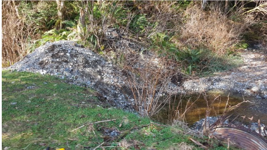
Photo 12 - Pile of dredged material from pool at Creek 3C inlet pipe
